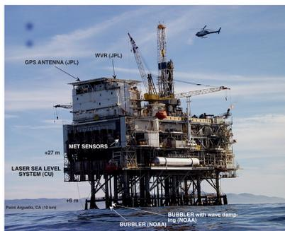
Figure 2: Arguello Inc. Platform Harvest, with locations of instruments that are being used to monitor the measurements taken by Jason-1 and TOPEX/POSEIDON.
