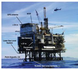
Harvest oil platform, equipped for altimeter calibration (from Haines et al., 2010)
