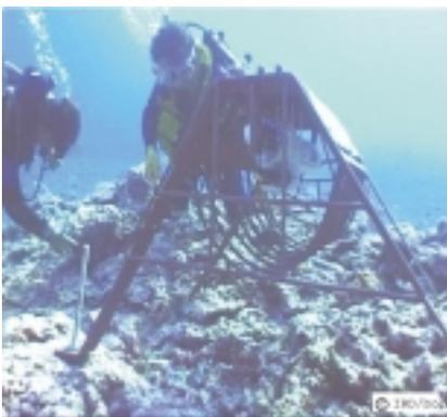
Figure 3: Tide gauge installation at Wusi by divers from IRD/Noumea. The device hosting the TG is designed in order that no mis-positioning can occur when the TG is removed and then fixed back for downloading/maintenance operations.
